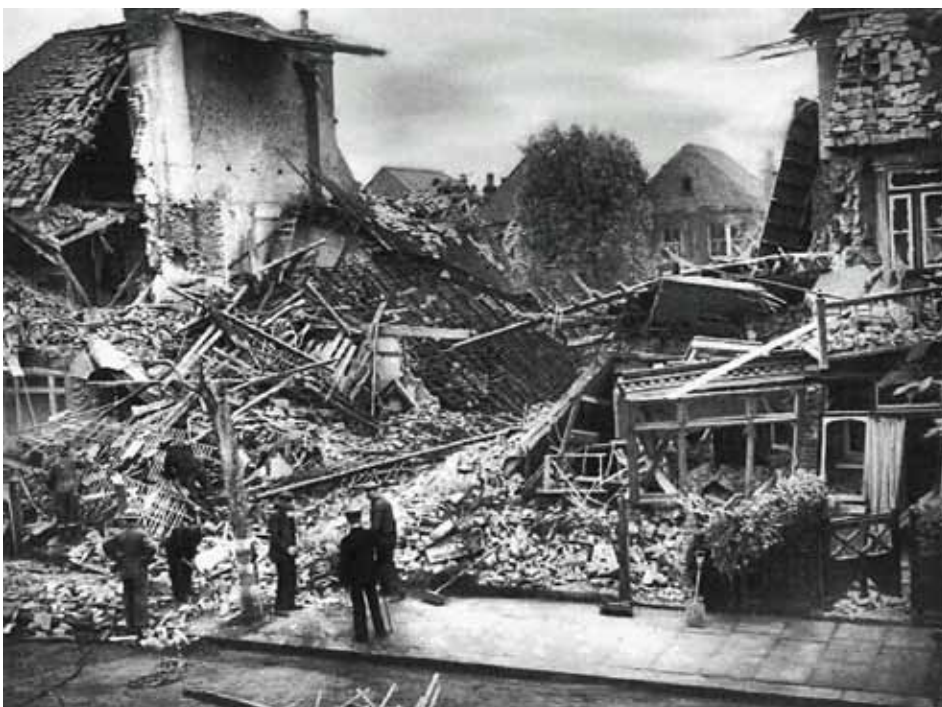
Damage done by V2 rocket in West Park Avenue
