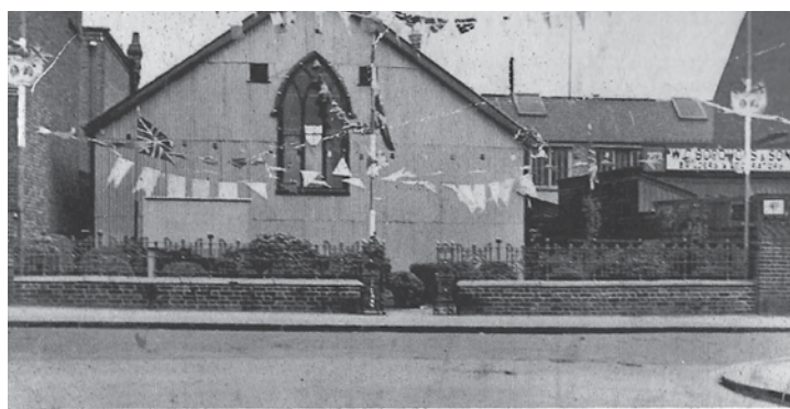
138 The Victoria Working Men's Club, with the original church window still in place.
